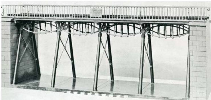
The first railway bridge in the world built by Stephenson on the Stockton - Darlington line in 1824
