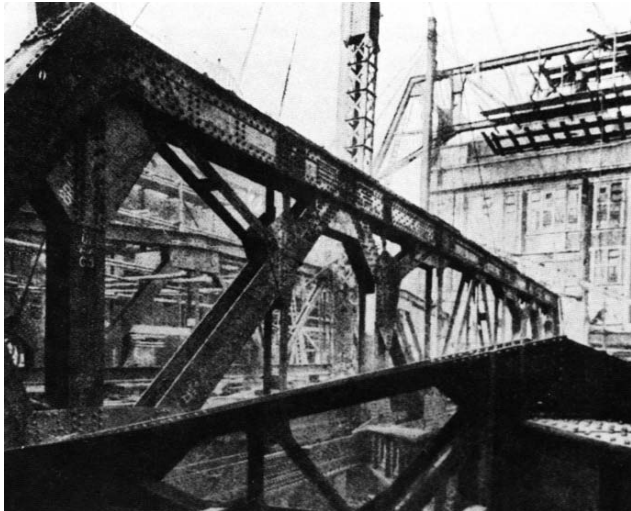
Cinema balcony girder
