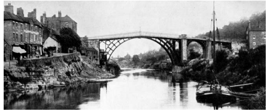
The first large span bridge in cast iron, Coalbrookdale, 1779
