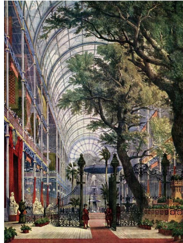
In the heydays of iron The Transept of the Great Exhibition of 1851. A striking example of the extensive application of iron for structural purposes. 3,800 tons of cast iron and 700 tons of wrought iron were used in the Exhibition pavilions
